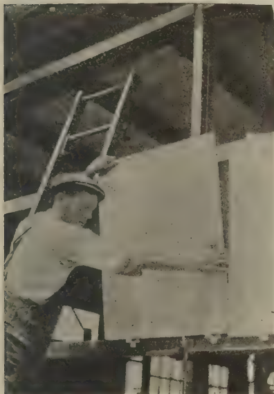
Note type of steel clip used to hold slabs in place
